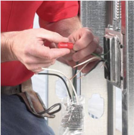
No time-consuming pigtails. Just connect the pre-stripped leads on the PlugTail connector.
